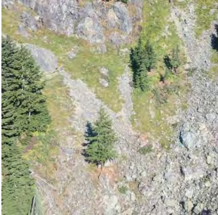
Figure 10 Aerial photo after improvement (Oct 4, 2017). Photo by Mike Lester.
